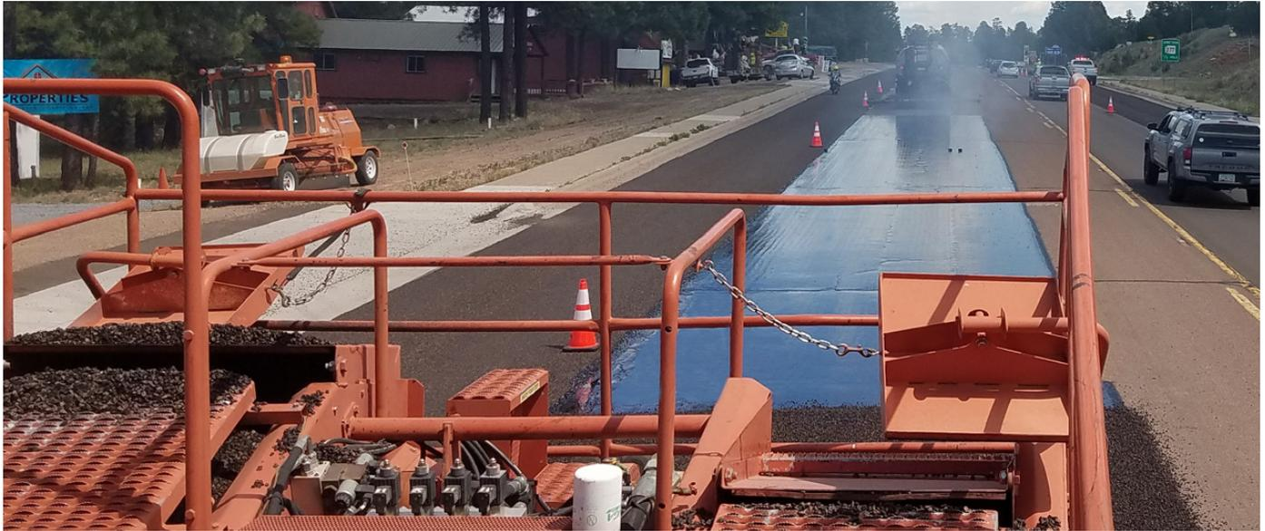
sealed, and a few small sections that were badly worn were milled and leveled. "ADOT needed to level the failed sections of SR-260 with the rest of the sections to assure rideability and safety," said Mo Rahman, PE, EAE West Region Technical Marketing Manager.
