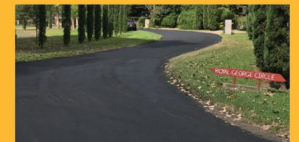
period of time due to heavy utility traffic, the distressed sections were cut out, replaced with new hot mix and compacted.
